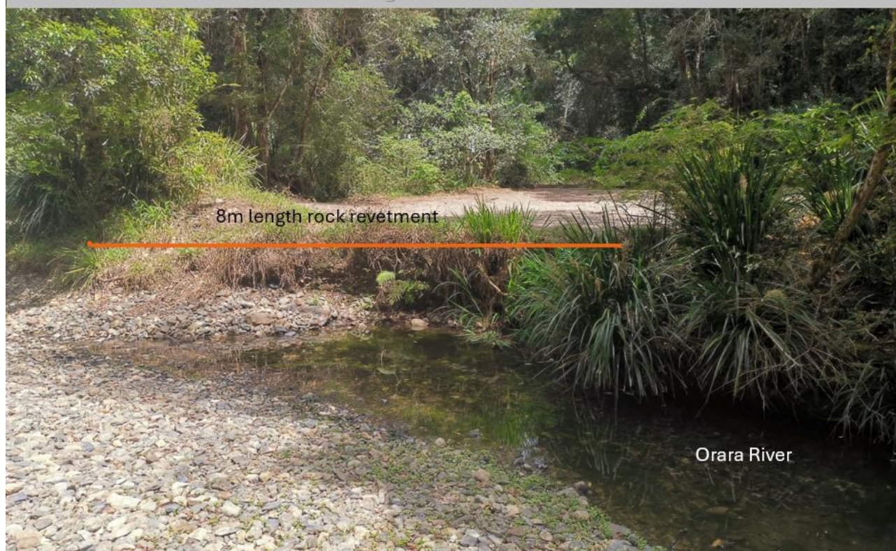
Site 1 – Rock revetment along 8m of eroded riverbank as per design by Shaun Morris of North Coast Local Land Services using 400-500mm rock
