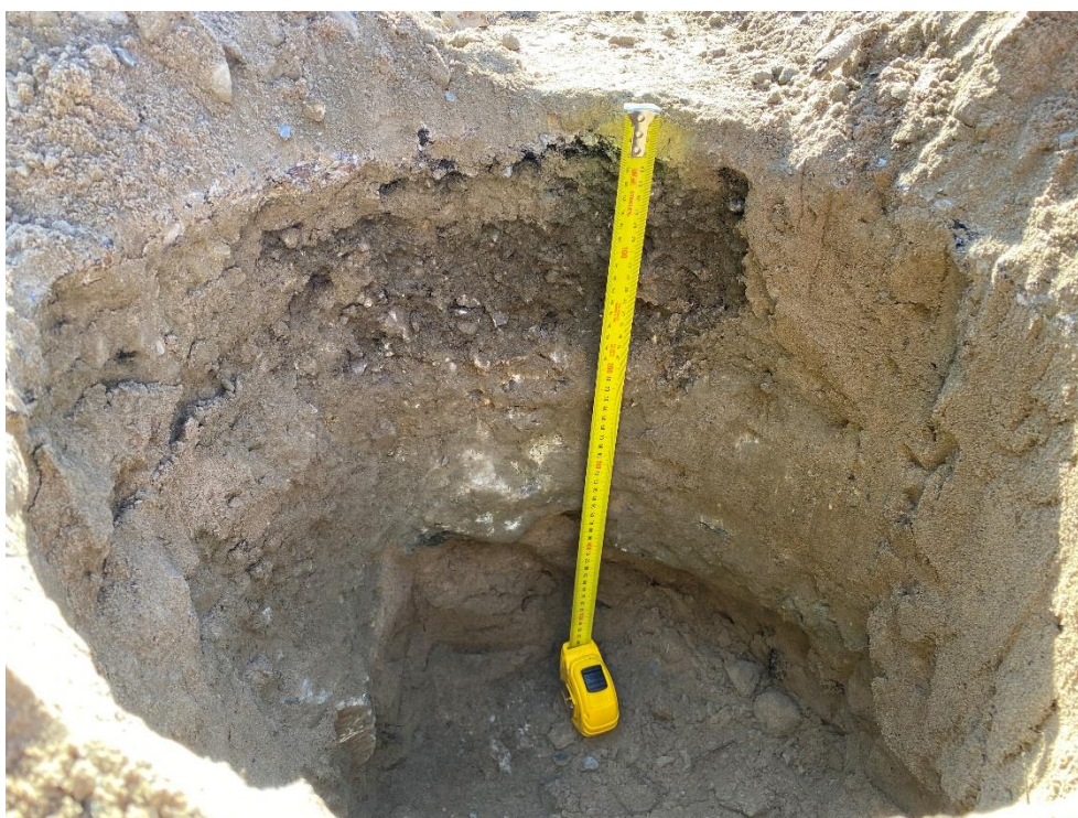
BH101 was typical of the materials encountered within the investigation and comprised a 40mm asphalt wearing course, over two pavement layers, over marine sand.
