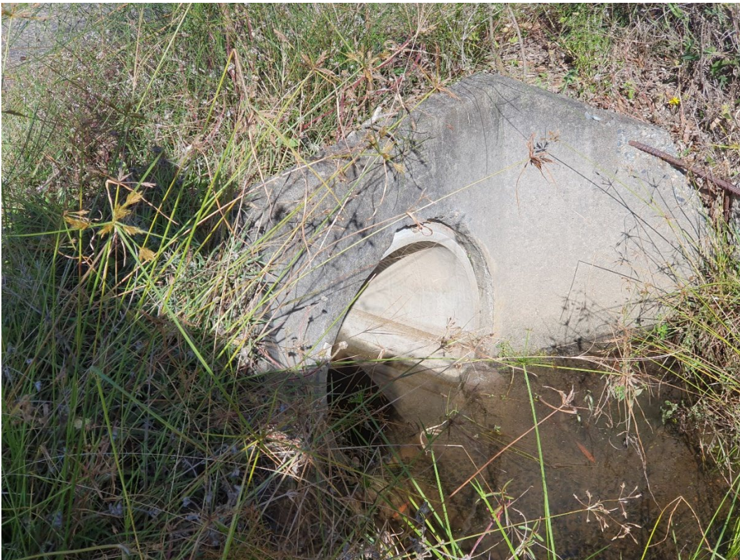
Plate 5.16 De Havilland Way culvert – water quality
