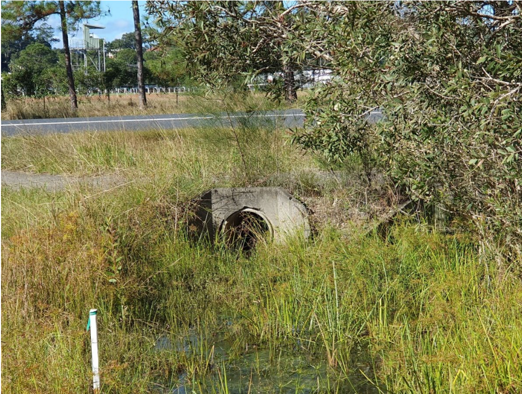
Plate 5.15 De Havilland Way Footpath Culvert - south side
