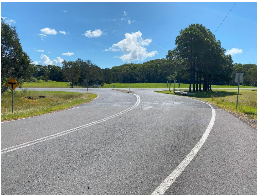
Looking west along De Haviland Way towards Hogbin Drive. The pavement level at the intersection is about 1m above surrounding surface levels.
