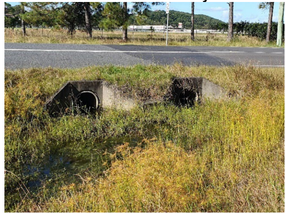
Plate 5.10 Existing culverts on north-west side of Hogbin Drive
