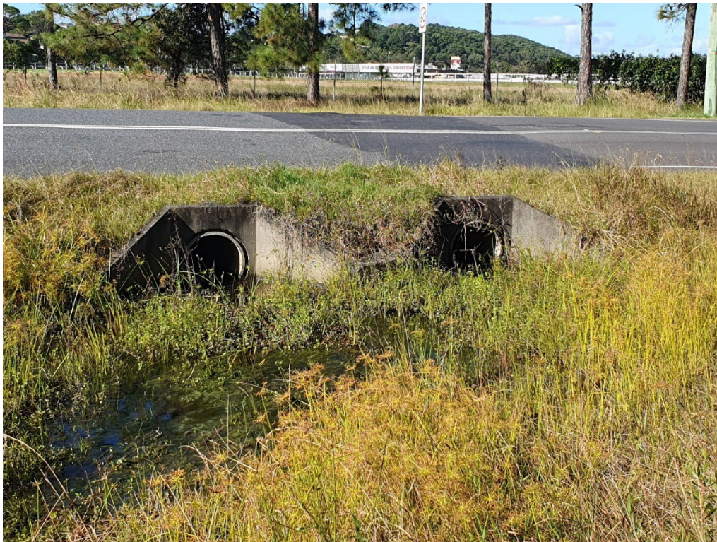
Plate 5.14 De Havilland Way Cross Drainage Culvert - south side
