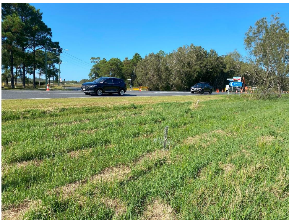
Looking southeast towards the existing intersection from the west of Hogbin Drive where widening is proposed for the roundabout and BH103 was drilled. Surface water was present on the day of the site investigation. To the west of Hogbin Drive, i.e. the grassed area, the site is underlain by marine clay.
