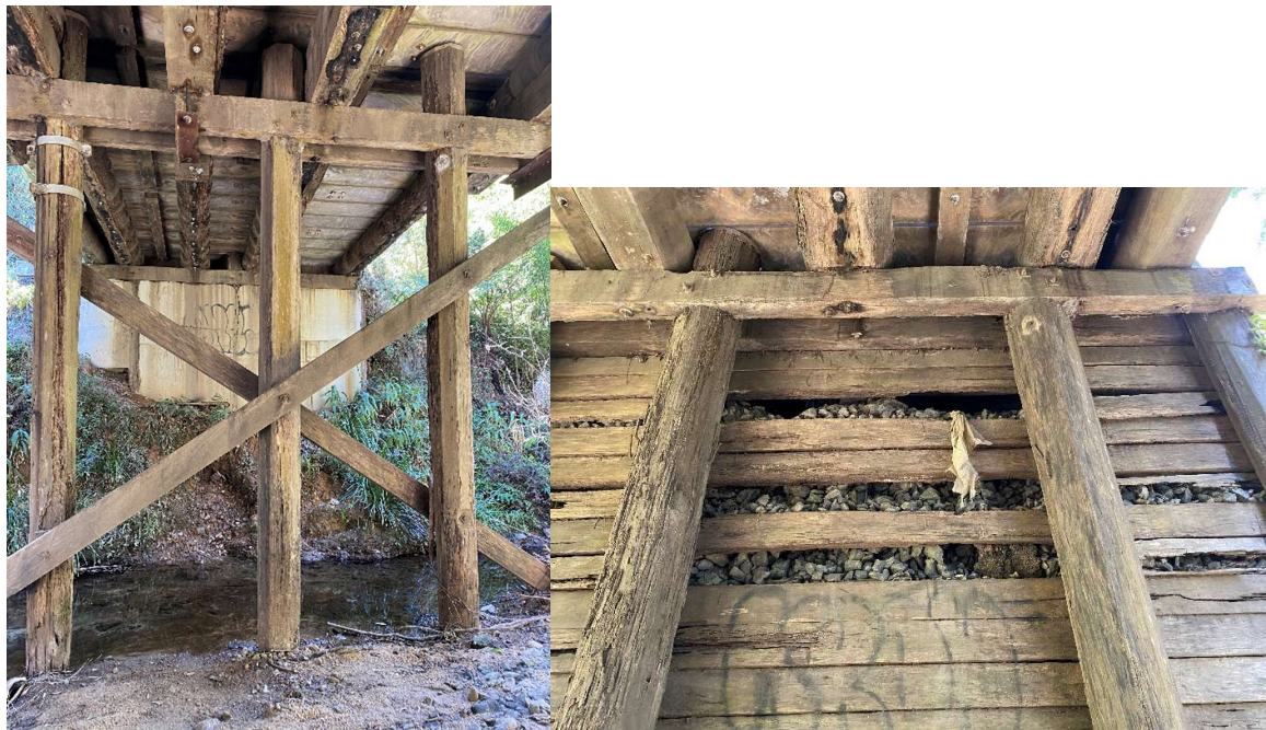
Figure 4: Examples of current condition of Bridge No.1
