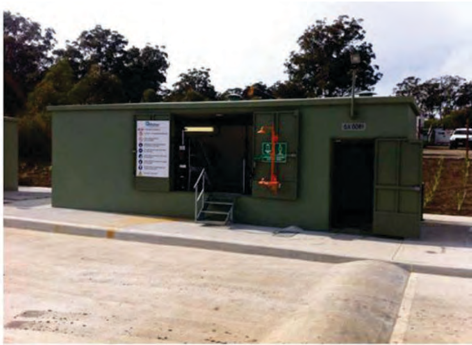
Sydney Water Corporation Chemical Dosing Unit -Appin
