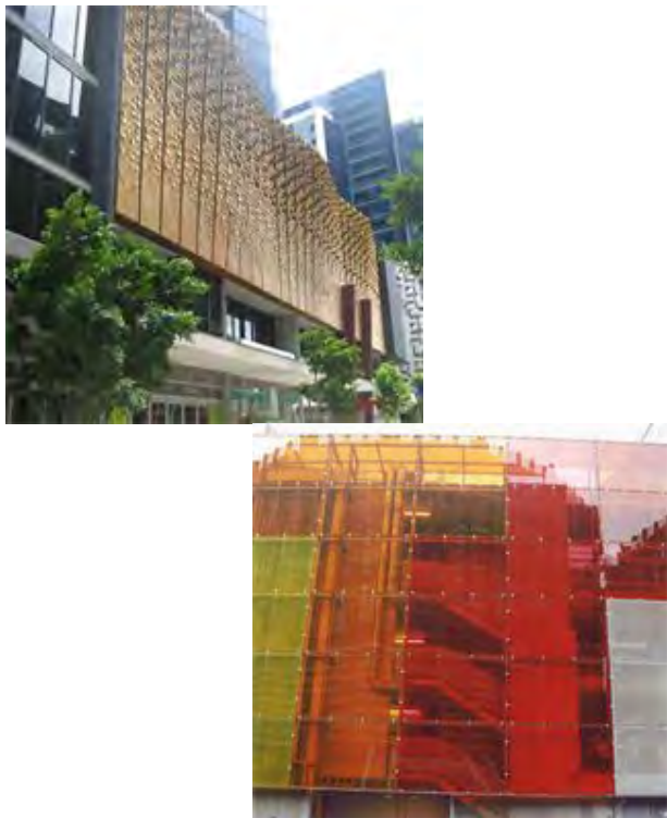
FIGURE 3 - EXAMPLES OF ABOVE GROUND PARKING OBSCURED FROM VIEW BY ARTWORK AND/OR SCREENING
