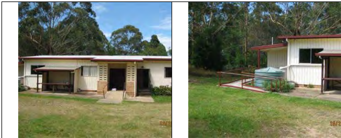
Eungai Creek community hall
