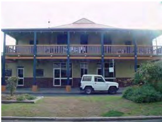
FIGURE 5 - SAWTELL HOTEL - C 1932 ONE OF SAWTELL'S MOST SIGNIFICANT HERITAGE BUILDINGS
